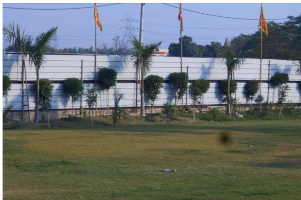
Figure 2.2 - Green Belt & Barracading around the project
