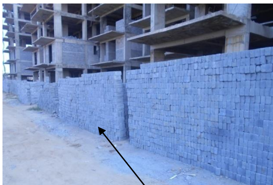
Figure 2.4- Use of Fly Ash bricks in construction
