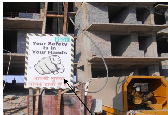
Figure 2.5 – Safety Boards at site
